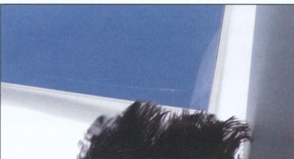
The walls of this skylight 40 feet high need to be cleaned with an extension pole and feather.
